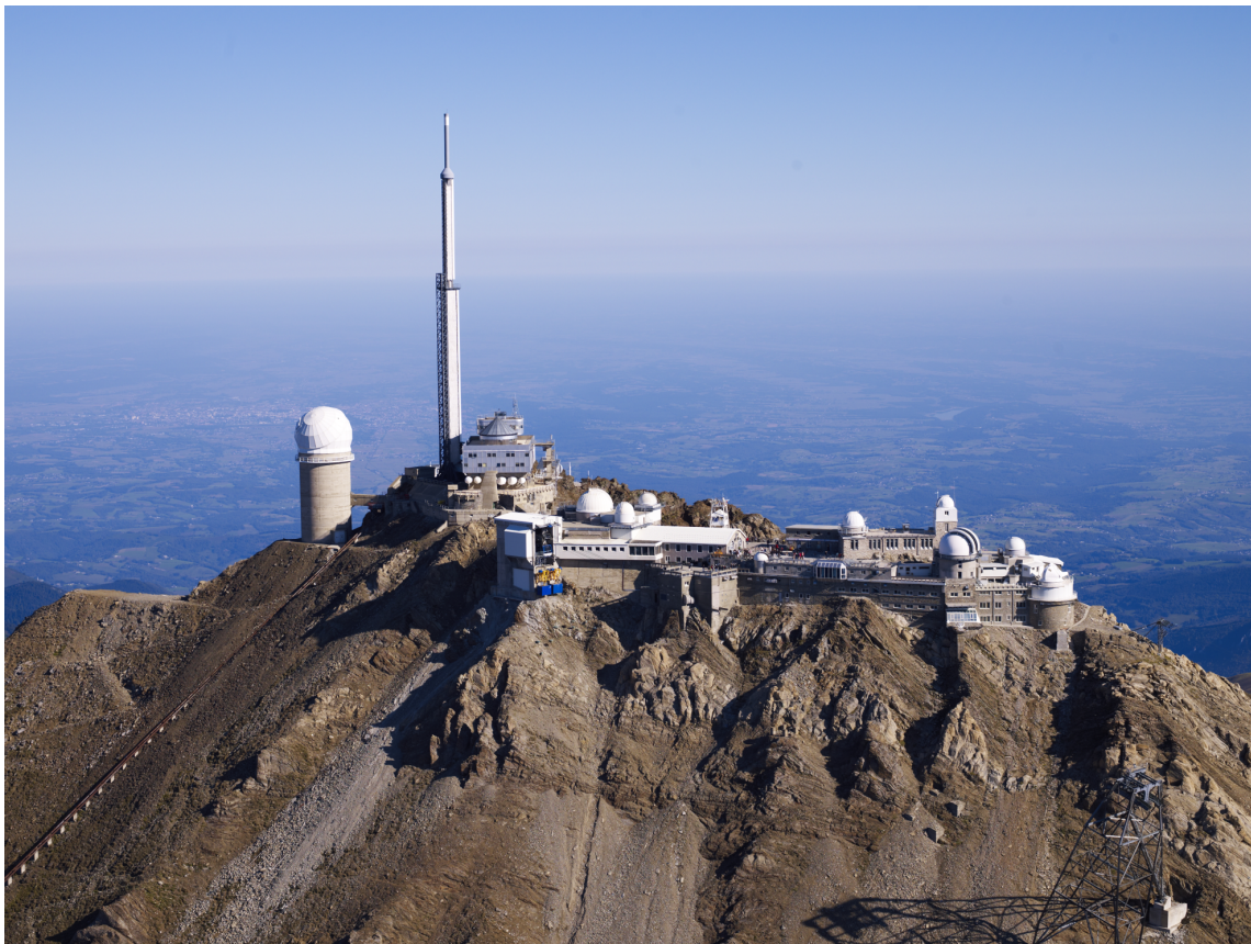
Fig. 9.6. Aerial view of the Observatory after the "Pic 2000" project in 2000. The new elements of infrastructure are visible: the cable car station, the footbridges, the new coronagraph building, and the modernising of the weather tower (2009). Photo © Claude Etchelecou
