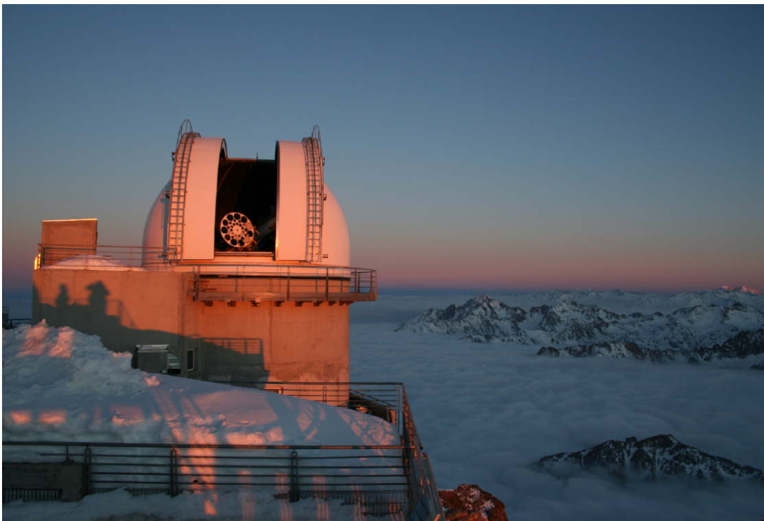
Fig. 9.41 The new dome and coronagraph ensuring continuous monitoring of the solar corona (2008). Photo © Régie du Pic du Midi and Observatoire Midi Pyrénées
