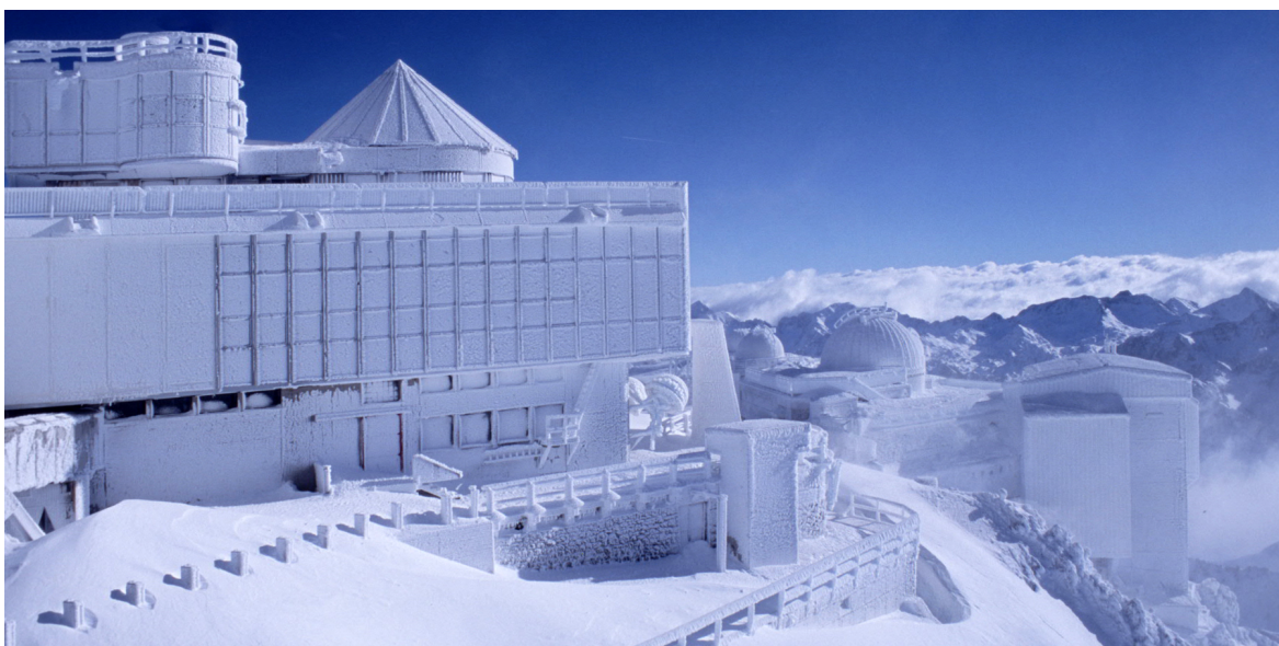
Fig. 9.42 Winter at the Pic du Midi. The buildings are imprisoned under the frost and the snow (2008). Photo © Nathalie Strippe
