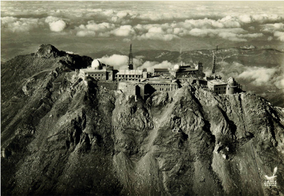
Fig. 9.35 Aerial view of the Observatory in 1960. The western part of the summit is not yet taken up with the interdepartmental building. In the centre, we can see the new cable car station at the top. Photo © La Pie servie aérien
