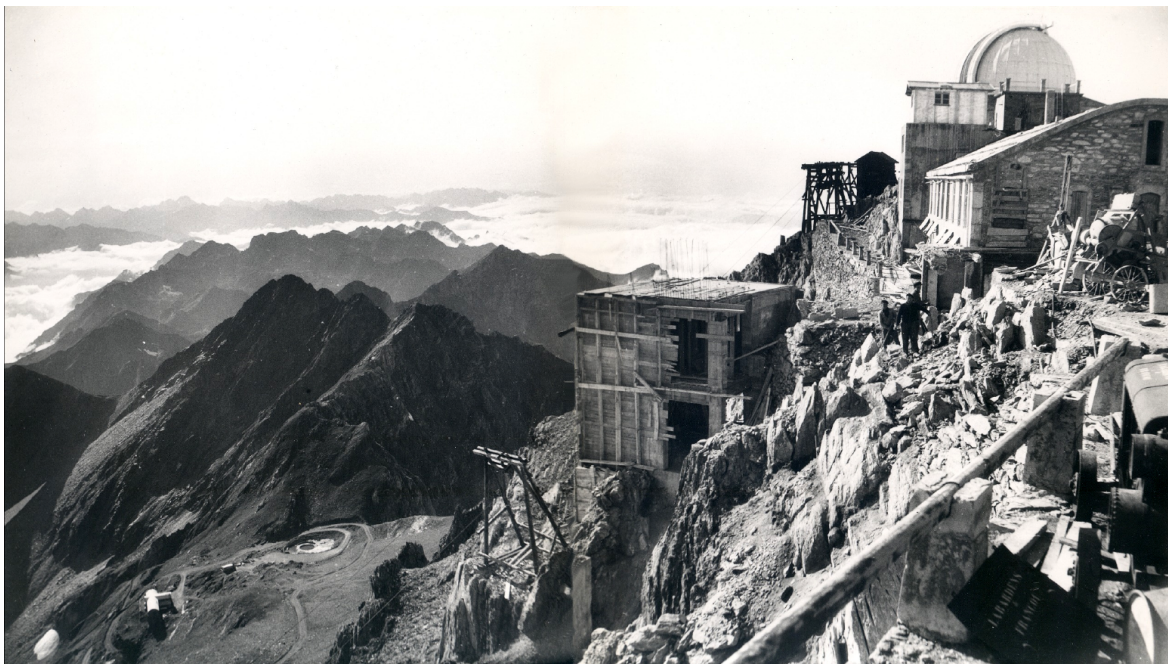
Fig. 9.33 Construction of the first cable car station on the south side of the Observatory, 1950. Photo © Alix, Fond Eyssalet
