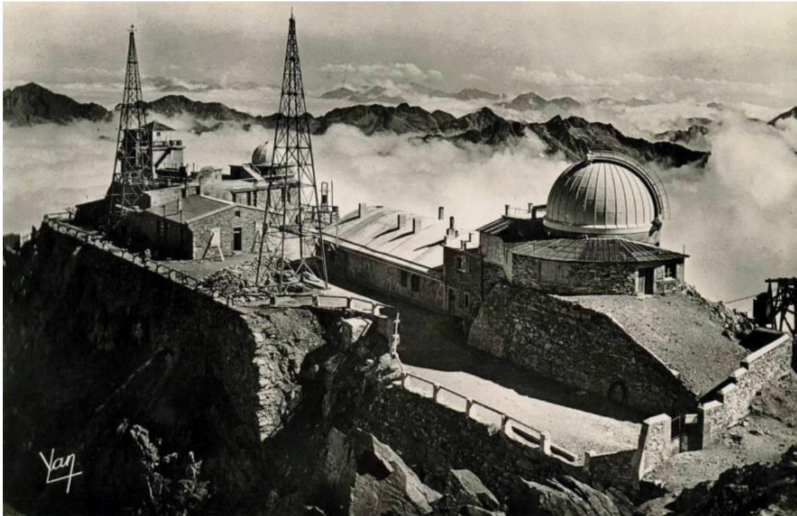
Fig. 9.32 The Pic du Midi Observatory in 1948. We can see the extension of the Dauzère building to the left of the image, the installation of the Gentili dome, and the Nanssouty building's new roof. Photo © Yan, Fond Eyssalet
