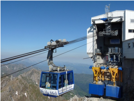
Fig. 9.39 The new cable-car station at the summit and the high-capacity cable car (2000). Photo © Régie du Pic du Midi and Observatoire Midi Pyrénées
