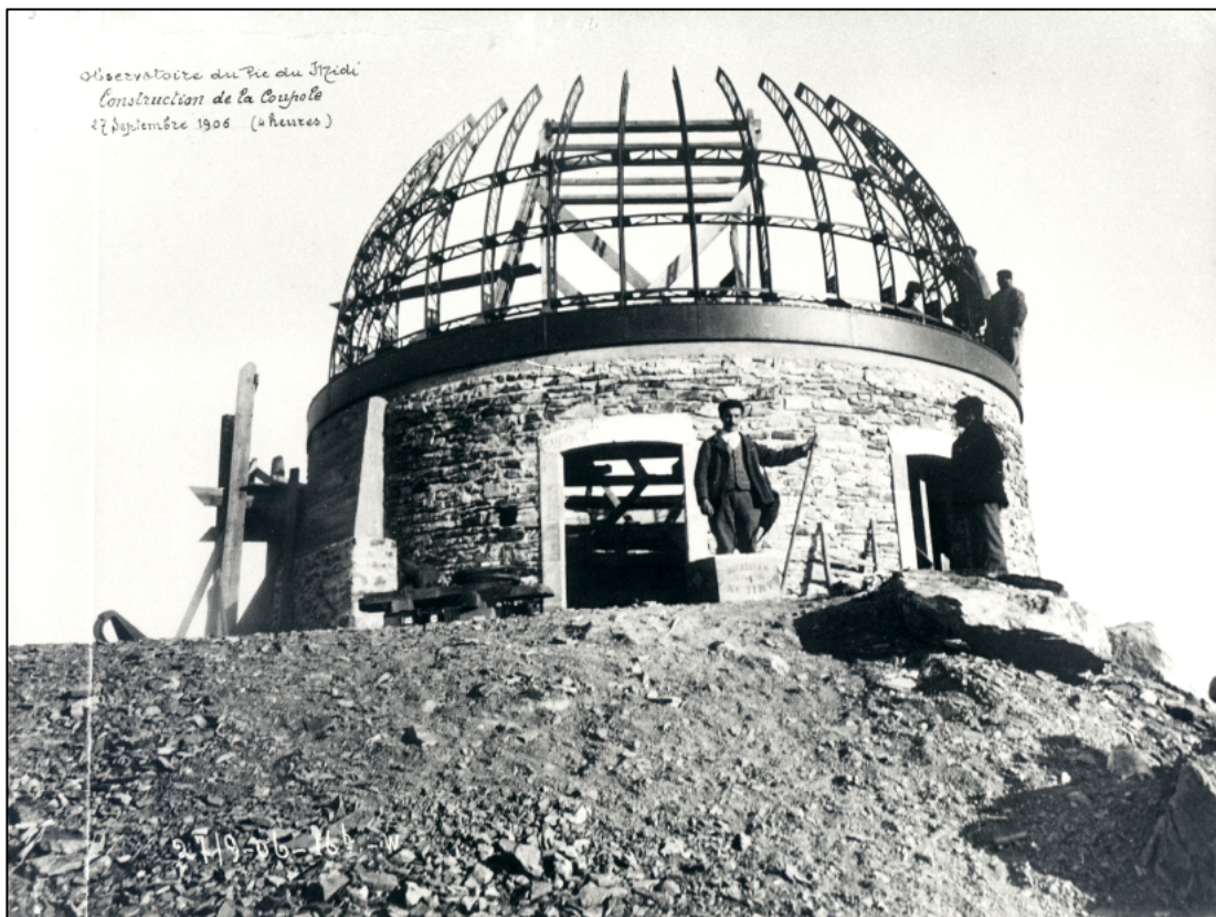
Fig. 9.7. Construction of the Baillaud Dome in 1907. Photo © Alix, Fond Eyssalet
