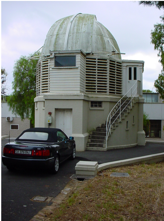
Fig. 8.6. Left: Helium dome with louvres for cooling and openable sides (1887). This dome houses the 18-inch reflector (1955), mounted on the original heliometer stand by Repsold. Photograph © Ian Glass. Right: Drawing of Helium dome as originally designed. Copyright © SAAO
