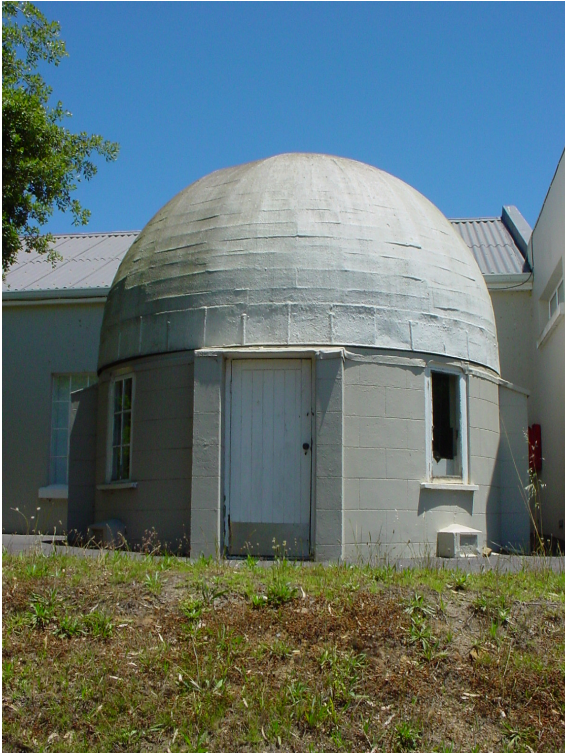
Fig. 8.5. Photoheliograph dome (1848). The wooden prefabricated dome, made in England, originally housed a Merz 7-inch telescope (1848) and now contains the De la Rue or Kew Pattern Photoheliograph made by Dallmeyer in 1875, mounted on a stand by Troughton and Simms (1874). Photograph © Ian Glass
