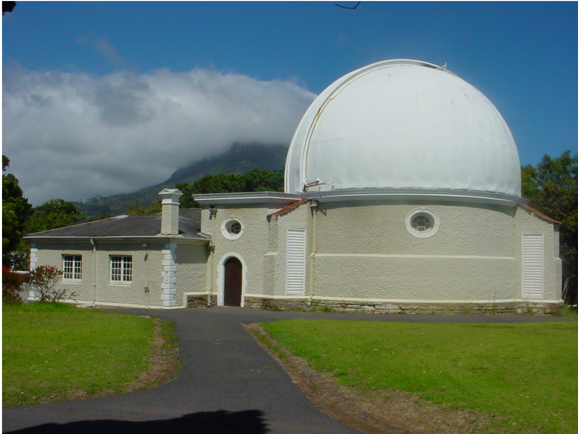
Fig. 8.3. Exterior of the McClean Building (dome and laboratory). Photograph © Ian Glass
