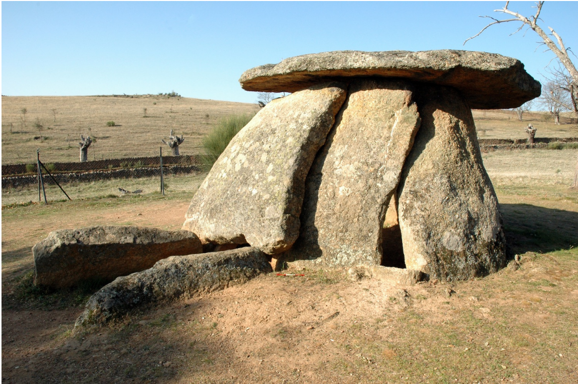
Fig. 3.5. Anta de la Marquesa, also known as Mellizo (no. 101 in Table 3.1), a good example of a short-corridor seven-stone anta with the addition of an eighth orthostat blocking the corridor. Photograph © Clive Ruggles
